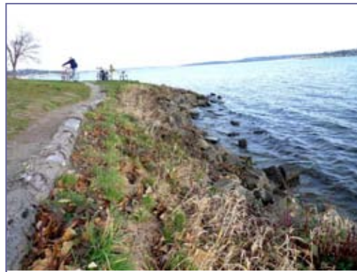
Concrete rubble shoreline armoring at Viewpoint 6
